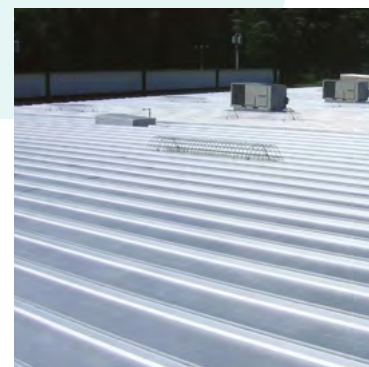
Step 3: Apply one coat of Alumanation 301
