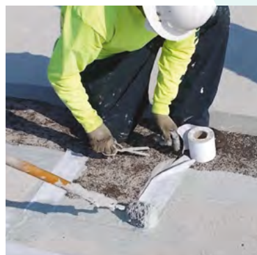
Step 2: Detail with the quick and easily installed seam sealer
