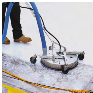
Step 1: Clean the surface of the metal roof
